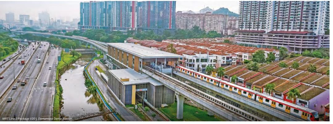
of 4.9 km of elevated viaduct including long span crossings over Keretapi Tanah Melayu (KTMB) tracks, and 3 elevated stations. The completion of the Putrajaya Line opens up further areas for development along its corridor and is set to be operational by 2021.
