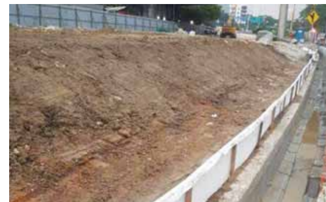
Silt Fence Installed As A Sediment and Erosion Control Measure
