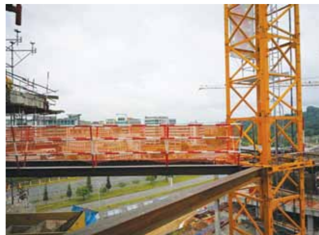
Fall Prevention Measures For Tower Crane Operators
