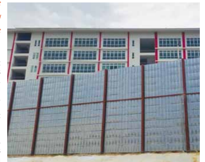
Noise Barrier Installed to Minimise Nuisance Caused by Our Activities
