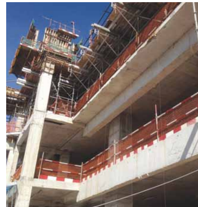
Edge Barricade As A Fall Prevention Measure
