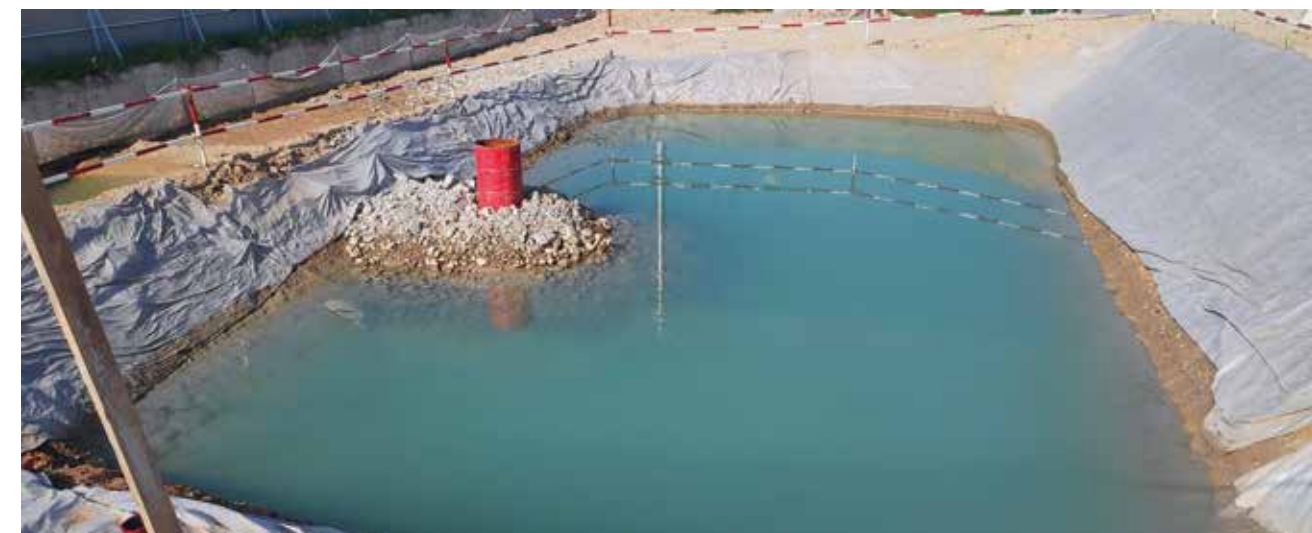
Silt trap for temporary containment of surface runoff to allow sedimentation before discharging
